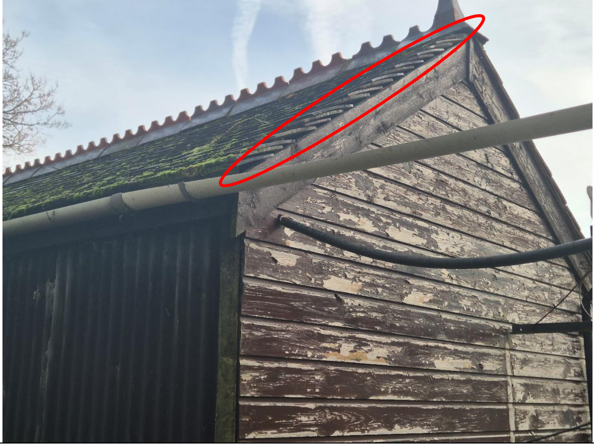
Gable end (south-west facing)
